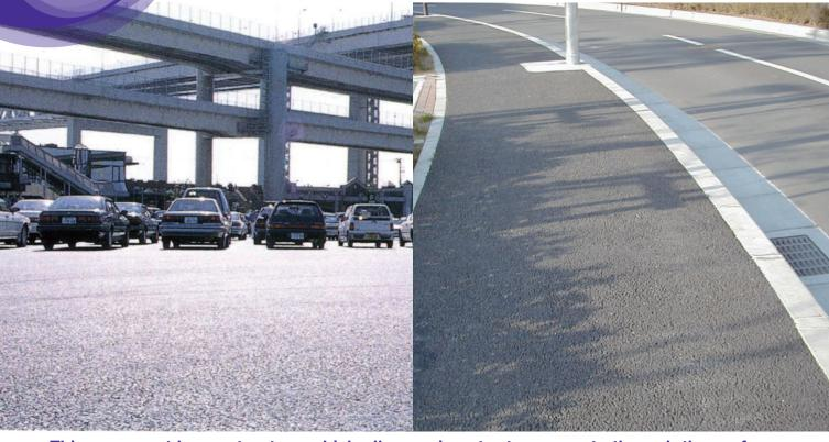
This pavement has a structure which allows rainwater to permeate through the surface course, the base course, and the subbase.
